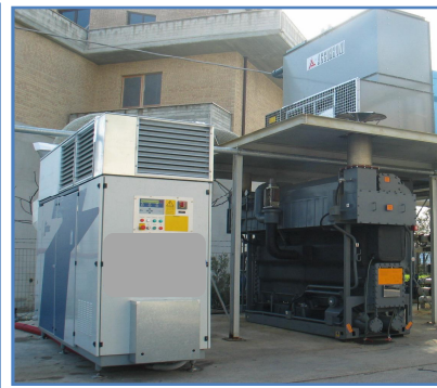
CCHP – cooling through hot water or exhaust gas
