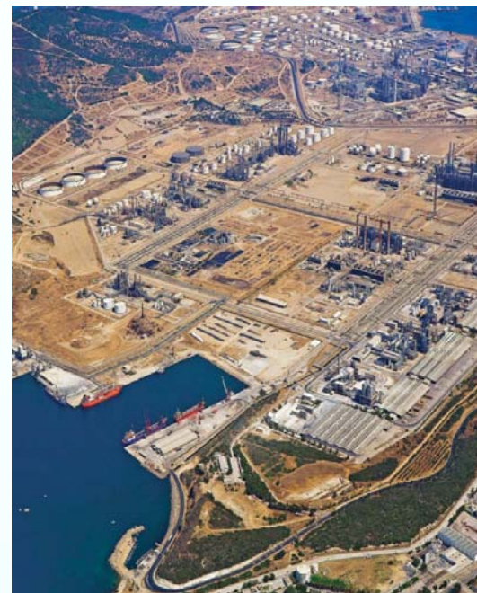
Aegean Refinery, Turkey
