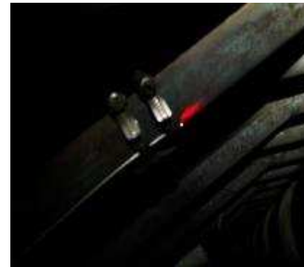
Fiber optic to measure temperature installed in HRSG header Unit 3
