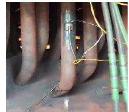
Skin point thermocouples installed in superheater header Unit 3
