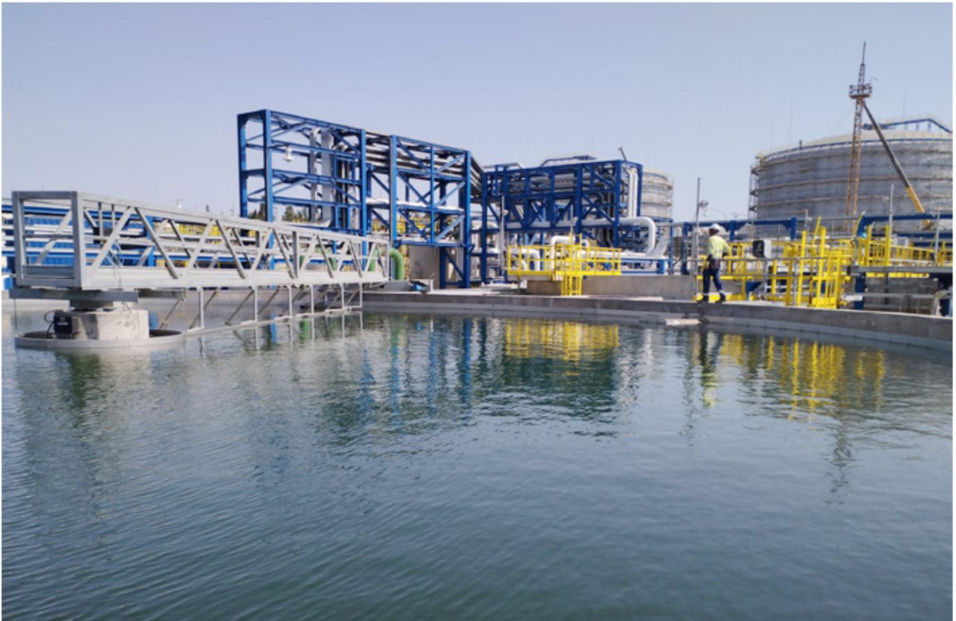
Alkaline chlorination: an optimized solution developed by Cannon Artes for cyanides reduction in a refinery water treatment plant
