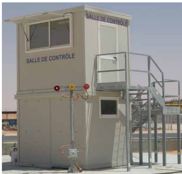
Fig. 8 - Control room for fire training ground
