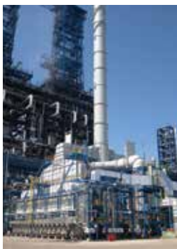
Terrace Wall™ heater for delayed coking unit, designed and supplied by Amec Foster Wheeler for Ufa Oil Refinery, Republic of Bashkortostan, Russia
