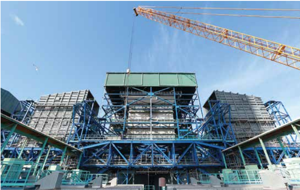
Erection of blocks connecting duct of Unit #2
