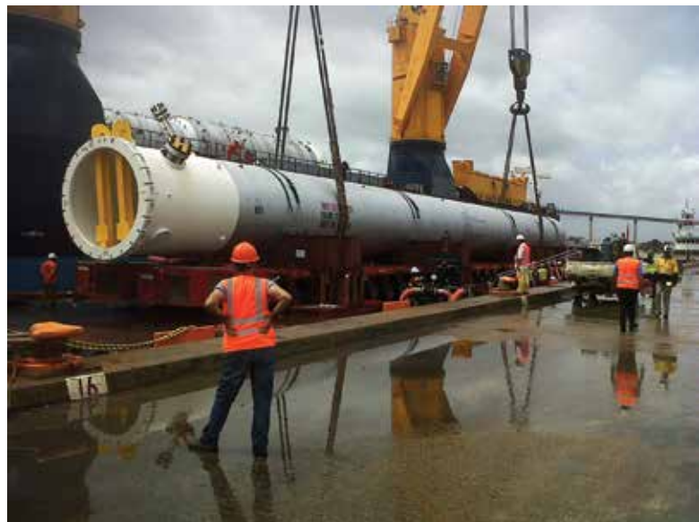
Fig. 14 - Direct unloading operations of heavy items onto the barge
