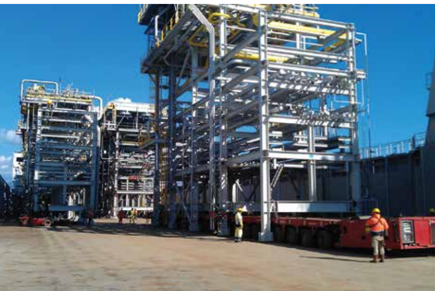
Fig. 3 - Load out of modules at Arbatax
