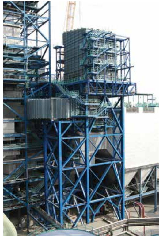
One SCR semi-block of DeNOx of Unit #2
