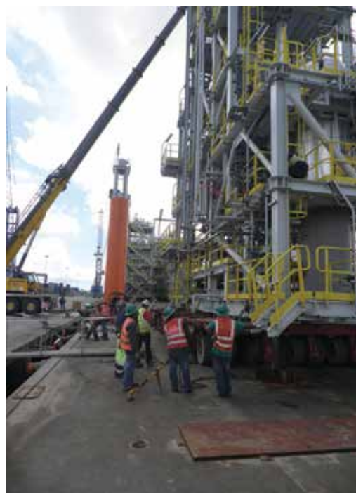
Fig. 16 - Direct load in ro-ro of modules onto the barge
