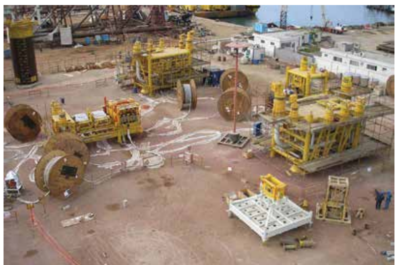
Fig. 5 - Subsea structures under construction that have been installed by Saipem in offshore Egypt (Burullus field)
