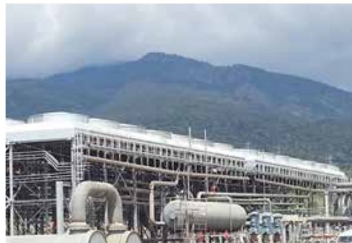
Fig. 9 - Spig air cooled condenser for geothermal binary plant
