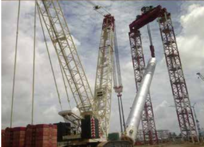
Fig. 28 - Installation with strand jacks and tower lift system
