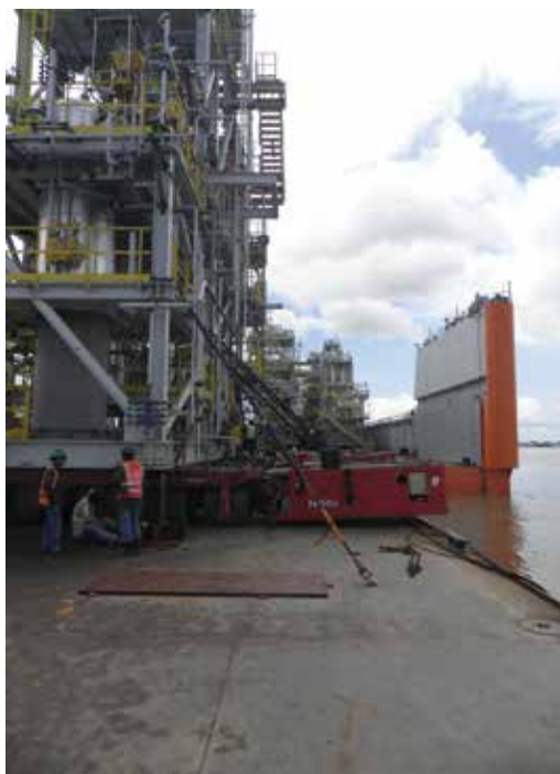
Fig. 15 - Direct load in ro-ro of modules onto the barge
