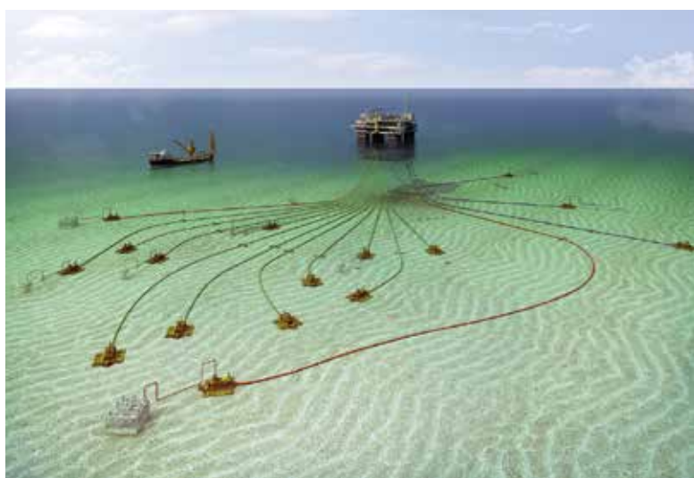
Fig. 3 - the P55 project executed by Saipem in Brazil (source: Petrobras)
