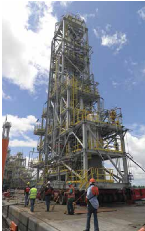
Fig. 17 – a) Transshipment phases of PAU 2604; b) transshipment from ship to barge of PAU 2064
