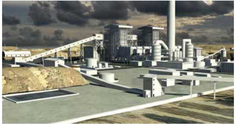
The view of the initial layout of the plant
