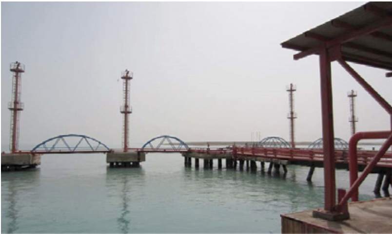
Series of remote controlled monitors employed for oil T-berth
