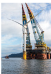
Ørjan Richardsen, Woldcam - Statoil - Mating of Hywind Scotland wind turbine
