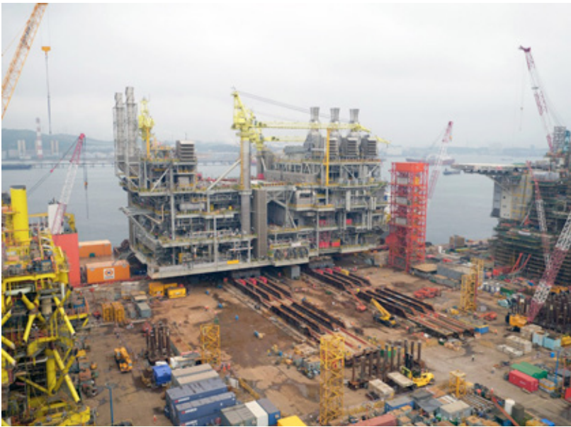
Skidding of the 44,000 ton section in Korea
