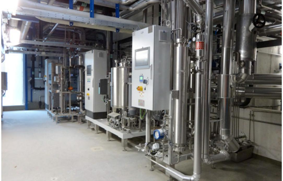
Fig. 5 - Technical Area with Pure Water Storage installation
