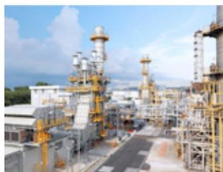
Modularised cogeneration plant integrated in a refinery complex, designed and built by Wood (formerly Amec Foster Wheeler) in Singapore, inaugurated in October 2017
