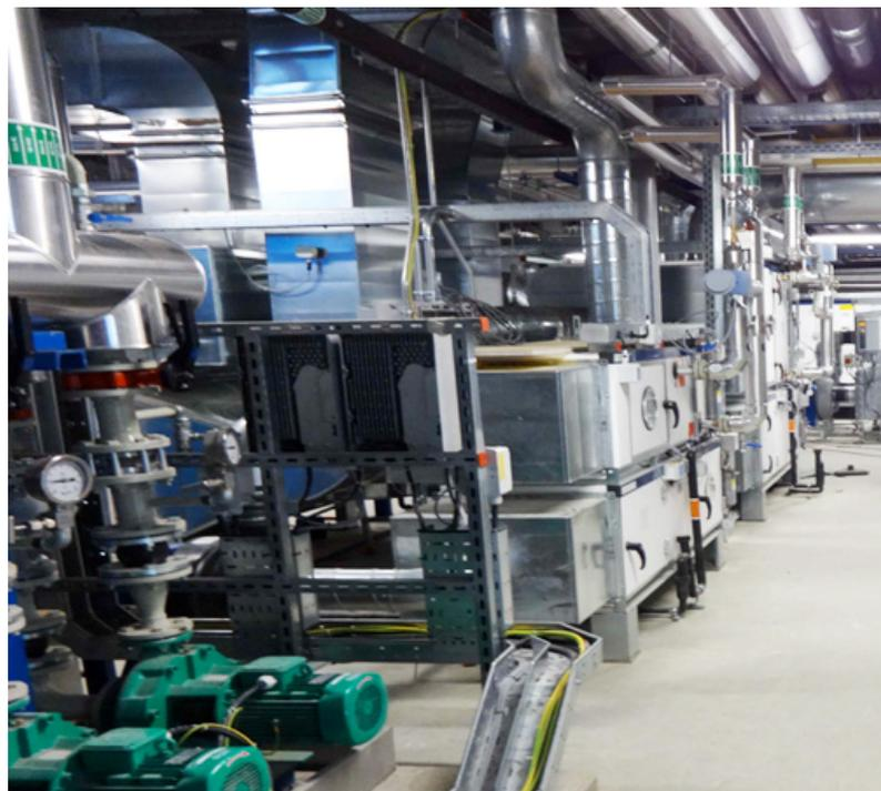
Fig. 4 - Technical Area with AHU (Air Handling Unit) installation
