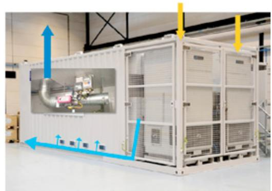
tion and the LER can operate as normal. Prolonged downtime and/or excessive wear is prevented by exchanging the units every eight hours. Each unit is equipped with a 100% backup fan and double compressors units are equipped with 2 x 50% redundancy on HVAC function.
