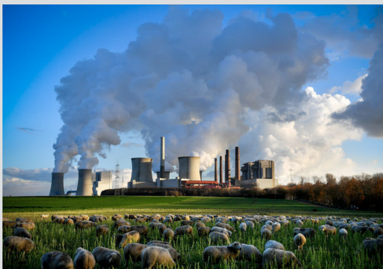
A traditional coal plant
