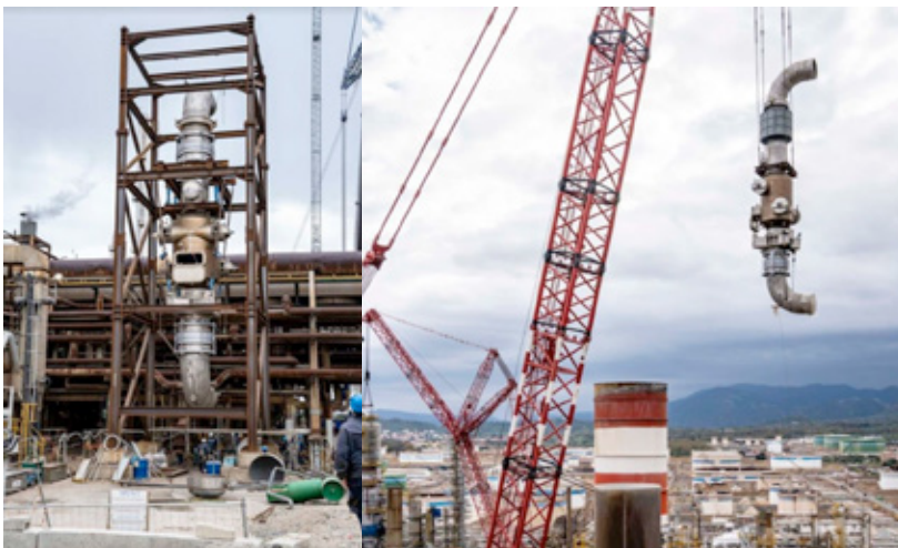
New isolation valve flue gas line module pre-assembly and lifting
