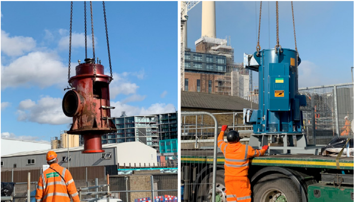
Removing the old pump's headworks - Courtesy of Stantec - IMAGE
