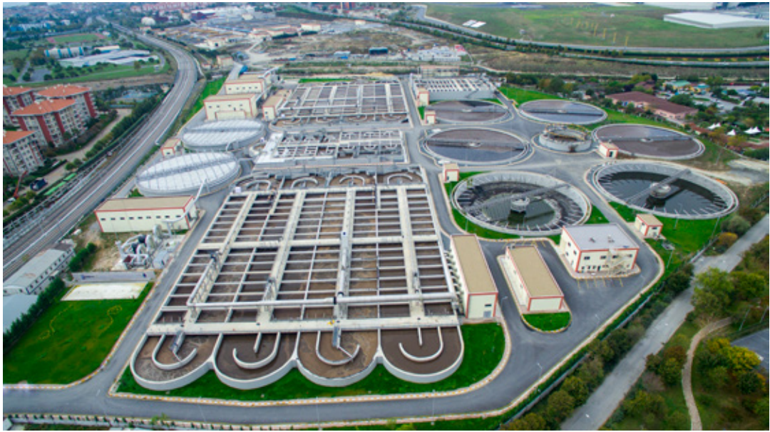
Atakoy Wwtp, Turkey (Fisia Italmimpianti & Alkatas). II Stage Main Plant
