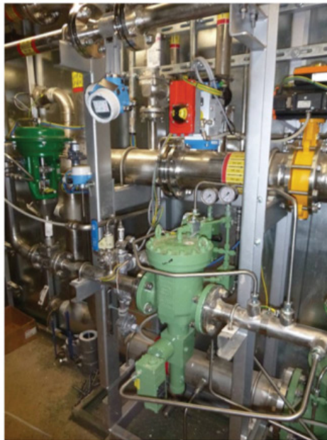
Figure 18: South Milford AD plant (UK) – Methane outlet
