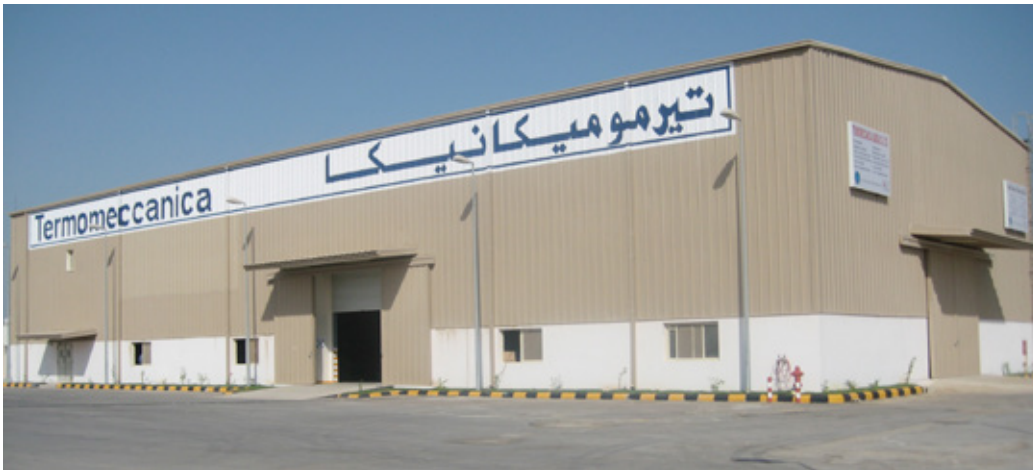
Termomeccanica Saudia workshop – outside view
