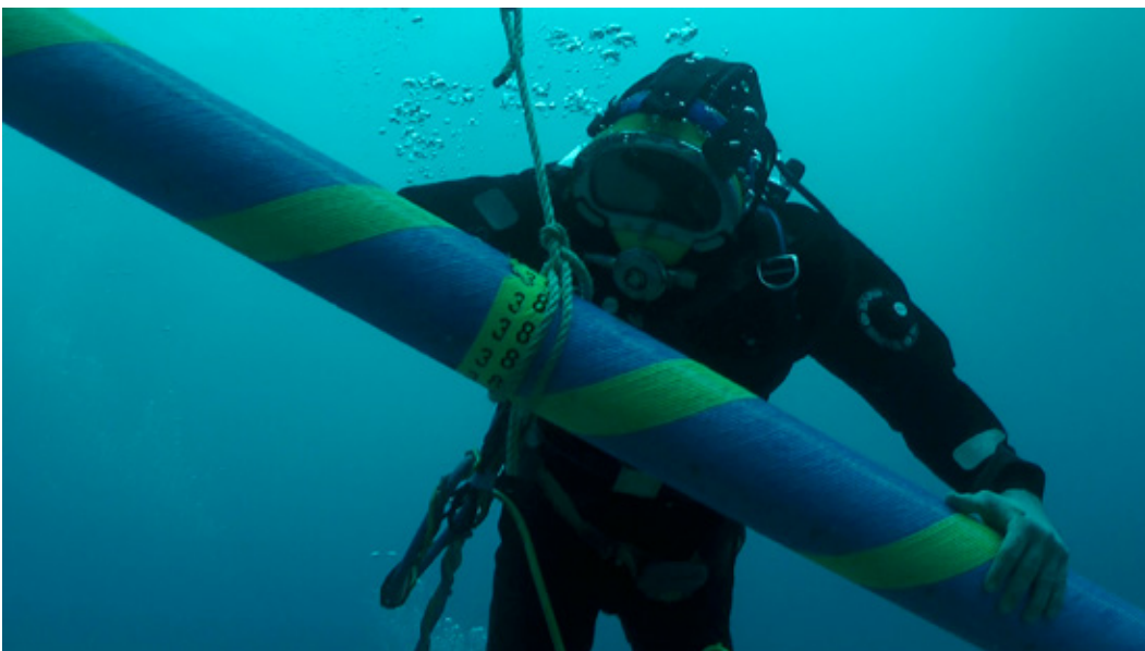
Submarine cable laying
