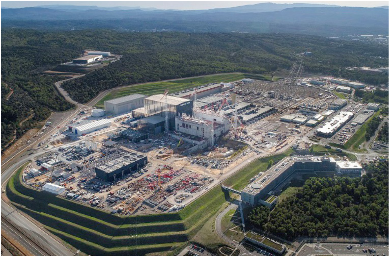
Tokamak building at Caradache - France
