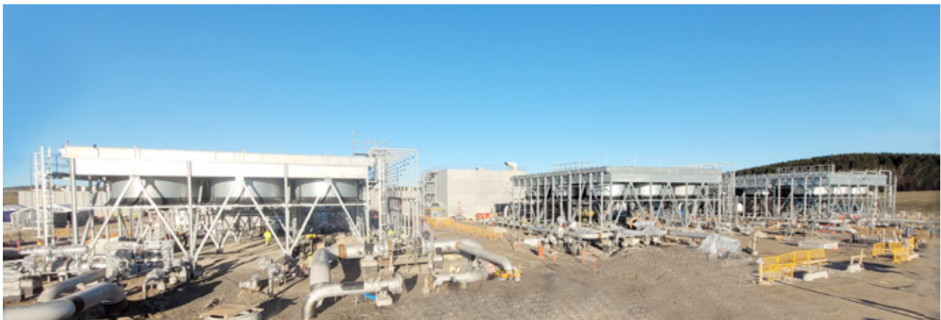
Figure 2: Ongoing assembly of the air coolers at site (Renco S.p.a.)
