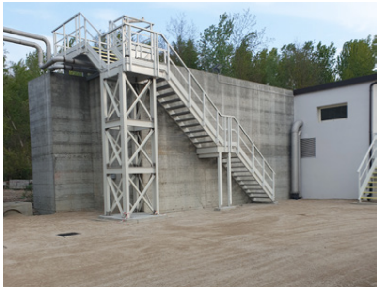
Constructing a FRP inclined stairway for tank access purposes
