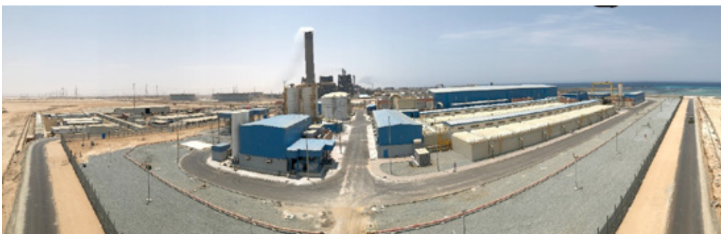
North West side panorama of Desalination plant in Shuaibah, Saudi Arabia (Fisia Italmimpianti & Abengoa)
