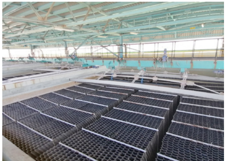
Dissolved Air Flotation system SALALAH IWP (Fisia Italmimpianti & Abengoa)
