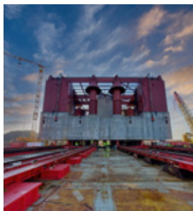
Denmark: load out of a 12,000 ton pylon foundation by means of 24 FAGIOLI skid shoes
